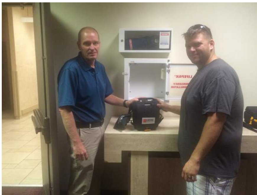
Scott Brauer (L) and Jason Caira (R) installing the new AED
